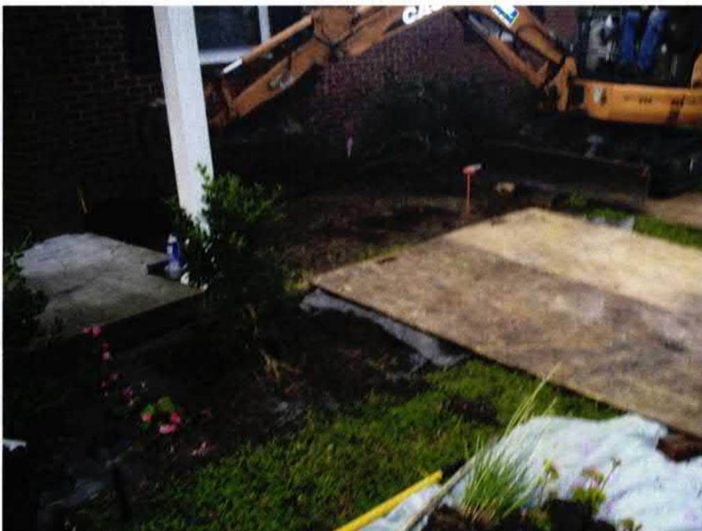
Picture 2: UST 1312Eagle removal in progress.
